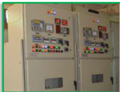
Indoor MV Switchgears upto 33 kV
